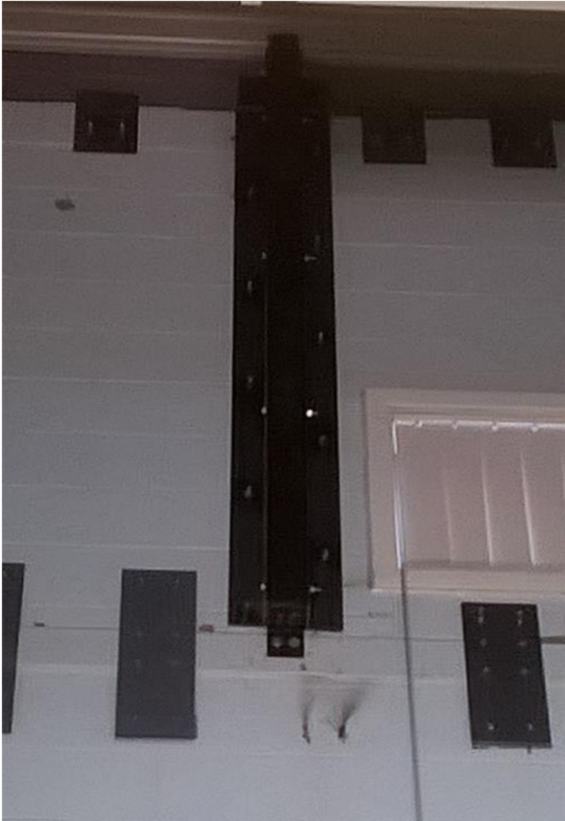
Image 18: Vertical windpost spanning from intermediate horizontal beam to roof beam and wall head restraints fitted to both beams as installed prior to boxing in and painting at Oxfangs School.
