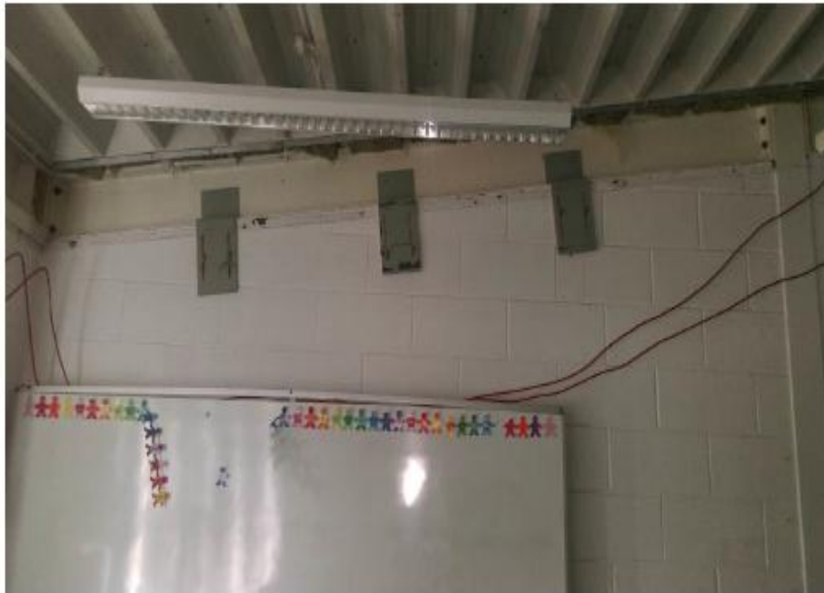
Room 059 – South Side (a)
