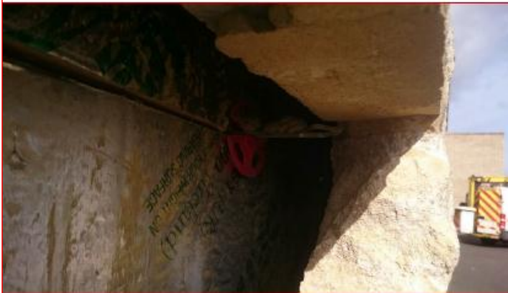
Photo 0187 Location 61B – Embedment 24mm
