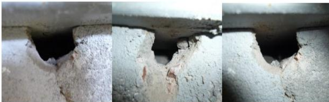
Image 14: Survey photographs demonstrating failure to find head restraints at Goodtrees Neighbourhood Centre.
