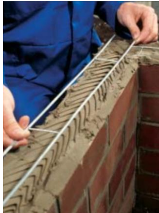
Image 25: Example of bed joint reinforcement
