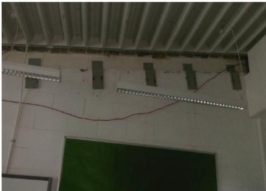
Room 059 – South Side (b)
