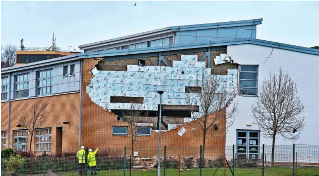
Image 2: Photograph taken at Oxgangs School of the gable wall after the collapse.
