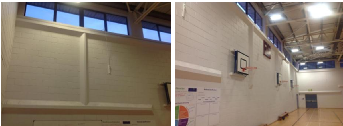
Images 19 and 20: Boxed in retrofitted windposts, Drummond High School.
